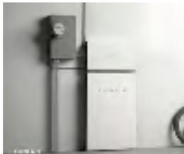
The Tesla Powerwalls collect and store solar power during the day and release it for use at night. In the event of an upcoming storm or hurricane, the Power Cells stop delivering electricity and retain even more energy to provide electricity when the electric lines are down. Most often, after a big storm, the day that follows is sunny, enabling the Powerwalls to be refilled.
