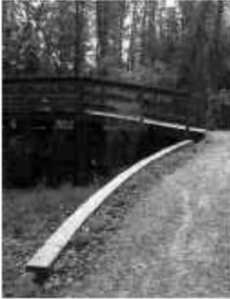
Approach to 2nd. Bridge #24&23
