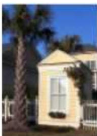
Jakes Lane Outbuilding #4
